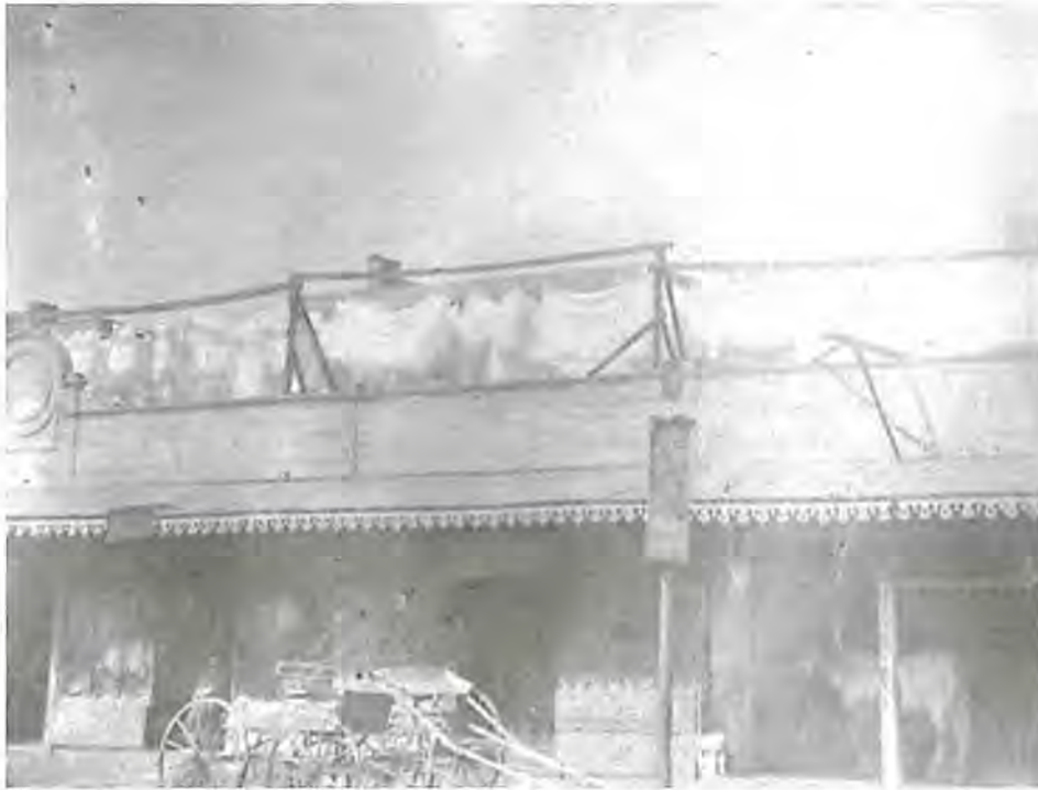
1. Photograph of the "Chinese Laundry House" of Yick Wo, 349 Third Street, San Francisco, showing wooden structure and roof-top drying lines, ca. 1885. Yick Wo was found guilty of violating a municipal ordinance that banned laundries in San Francisco unless lodged in brick buildings. He filed for Habeas Corpus in the San Francisco U.S. Circuit Court. In overturning his conviction in 1886, U.S. Supreme Court affirmed the opinion of the latter, that discriminatory enforcement of the ordinance deprived him of "Due Process" under the 14 th Amendment.
