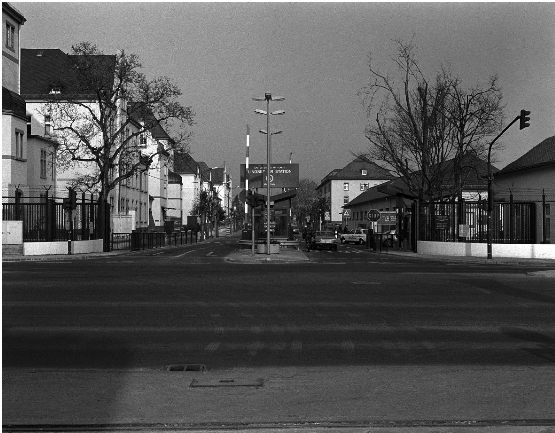
Recently renovated front gate, 4/15/1987, Lindsey Air Station, Wiesbaden, West Germany (FRG)
