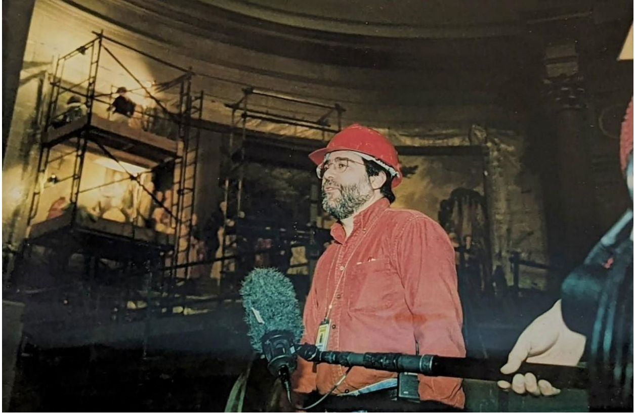
Rick Blondo in the National Archives Rotunda during renovations, circa 2002.
