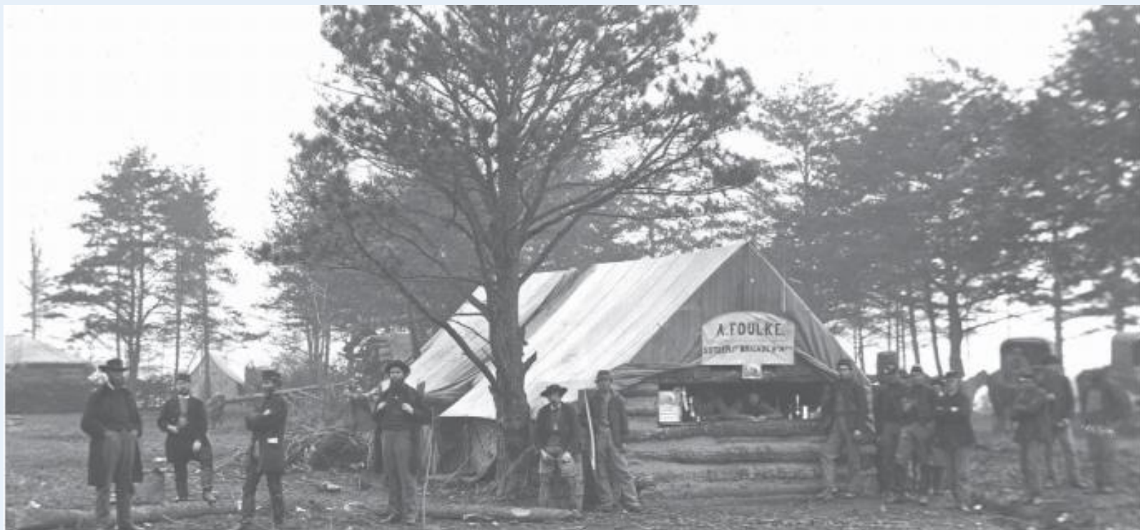
Tent of A. Foulke, Sutler, at headquarters of 1st Brigade, Horse Artillery, Brandy Station, Virginia, February 1864. Photograph by James Gibson. LC-B817-7165. Courtesy Library of Congress. Online: http://www.loc.gov/pictures/item/cwp2003000260/PP/ . Foulke is the fourth man from the left. The tent's sides are made from logs due to the semi-permanent nature of winter quarters, which lasted from December 1863 to April 1864. For more about Foulke, see Marlan H. Polhemus, "'A. Foulke, 1864,' Tracing a Civil War Inscription," American Society of Arms Collectors Bulletin 85 (2002): 25–33.
